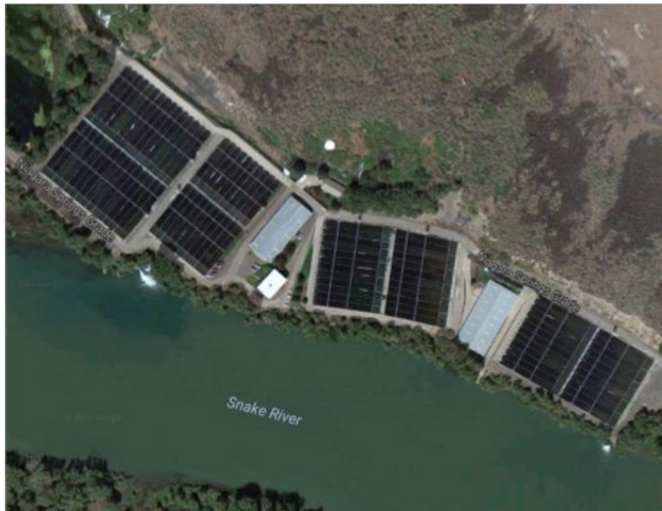
Figure 6: Aerial image of a large trout farm in the Hagerman Valley, Idaho. Note the discharges (whitewater) into the Snake River, whereas the raceways are surrounded by concrete.
